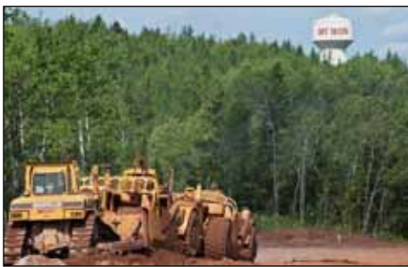
Site work is underway at the Mountain Iron Renewable Energy Park.
